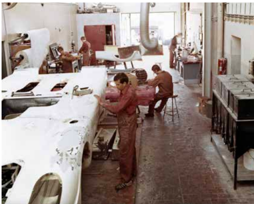
Production of the body of the 917 in 1969 at factory 1 in Zuffenhausen
