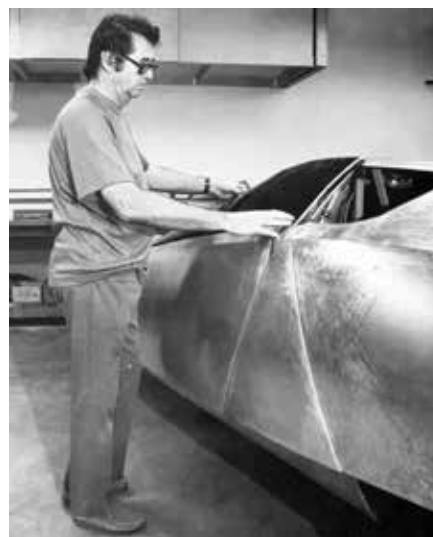
The sheer lines mandated by Pelly’s design made heavy demands on the skill of Dick Troutman. Working to a wooden buck, he succeeded in manipulating its aluminum.
